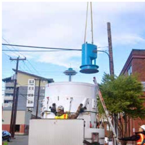
**Loading a research irradiator into the 10-160 B package.**
