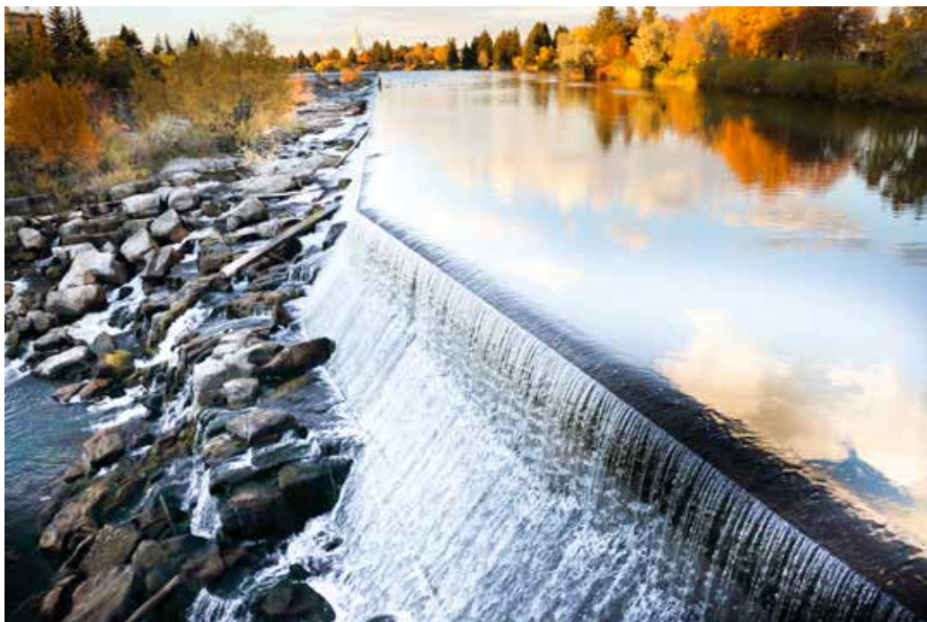
Idaho Falls Power, a collaborator on the project, has four ROR power plants on the Snake River. Here, a diversion dam directs much of the water toward a nearby hydro plant. (Photo courtesy Idaho Falls Power)
