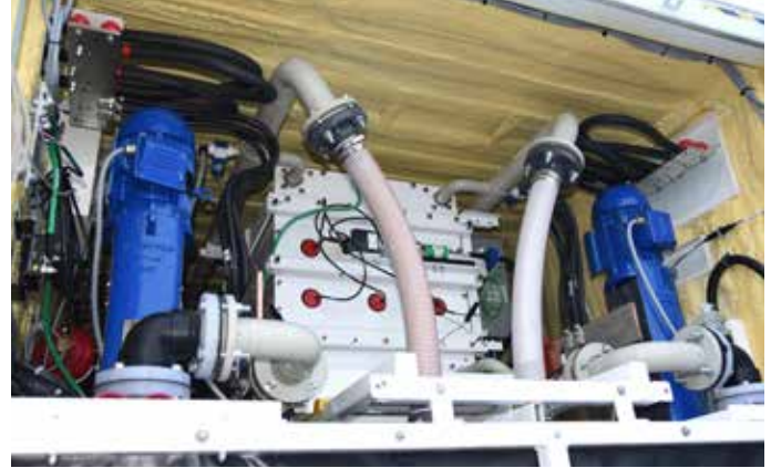
Each flow battery includes four fuel stacks in which the energy generation from the ion exchange takes place.
