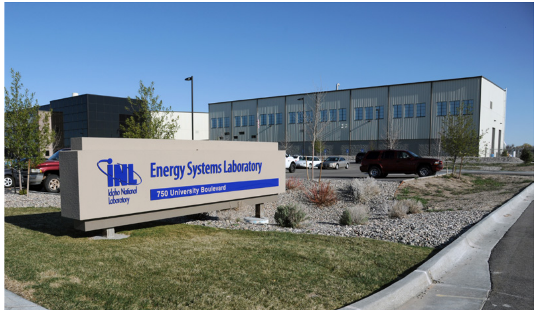
INL's Energy & Environment Science and Technology Directorate added a 91,000-square-foot testing and demonstration facility called the Energy Systems Laboratory (ESL) in 2012.
