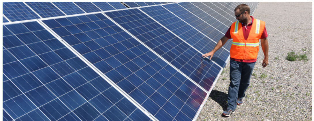
INL energy system testing integrates a renewable energy microgrid with load-control, simulation and storage capabilities.
