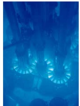
*ATR's core overhaul process renews the reactor by replacing components nearest to the core (shown in blue). Those components experience the heaviest long-term wear, particularly the reflector blocks (shown in red).*
